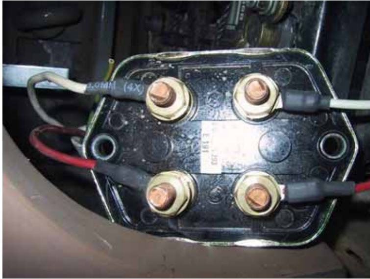
Figure 10 Isolation Switch Connections
