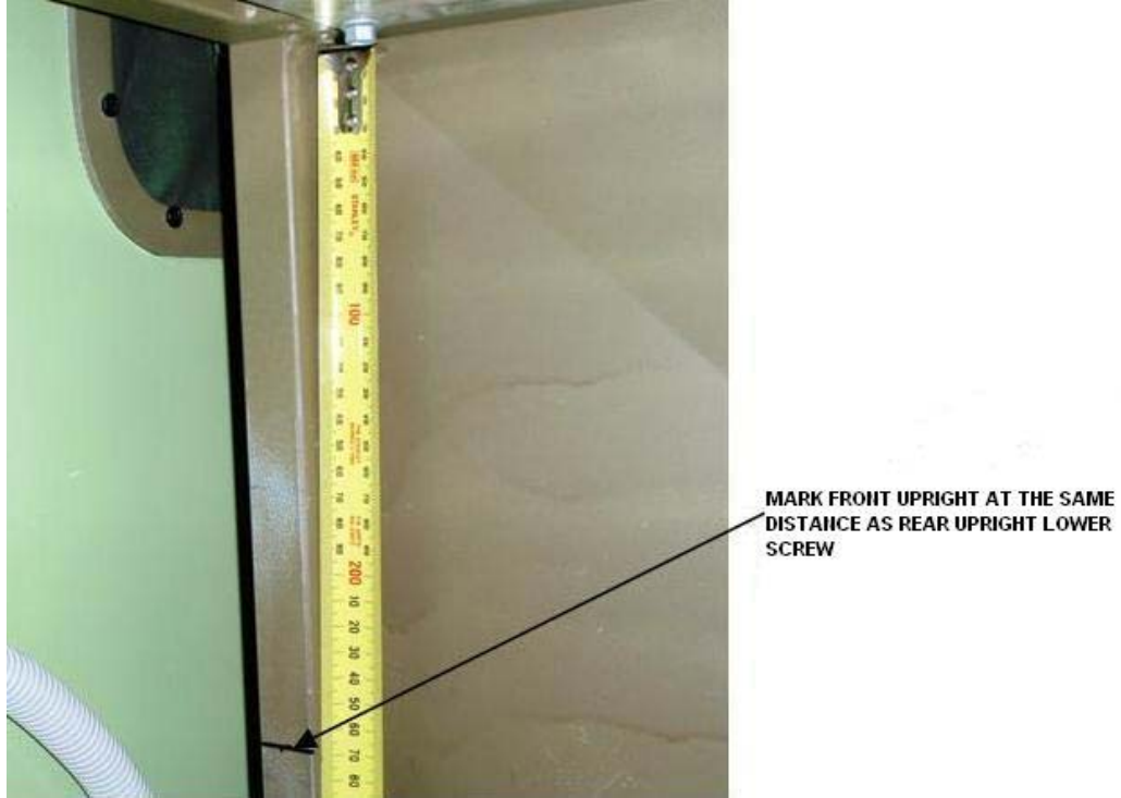
Figure 7 Marking Front Upright Support Post
