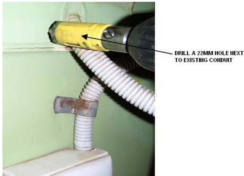
Figure 10 Drill 22 mm Hole
