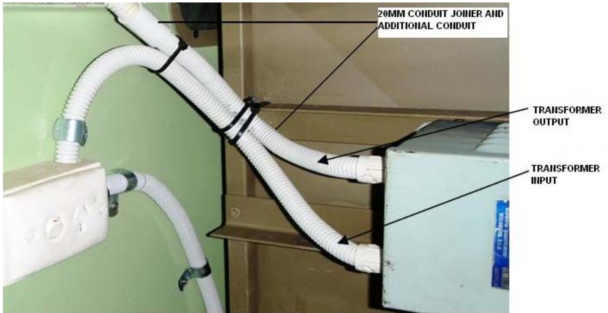
Figure 9 Transformer Final Assembly Position
