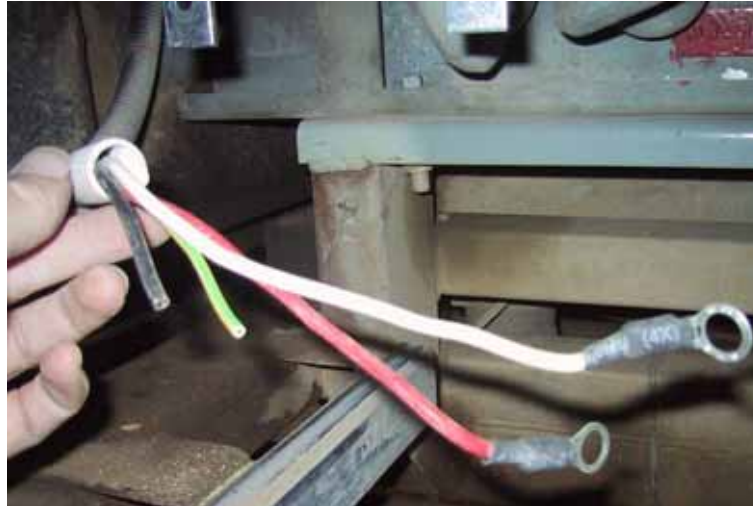
Figure 14 Module Wiring To Switch Connection Points
