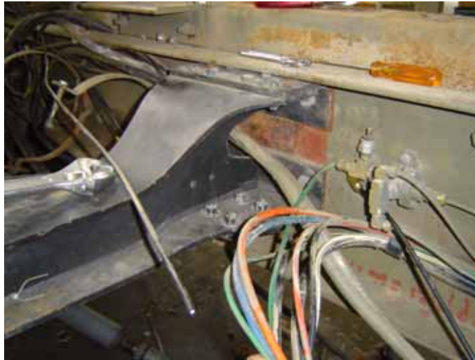
Figure 12 Tying Back Air Lines
