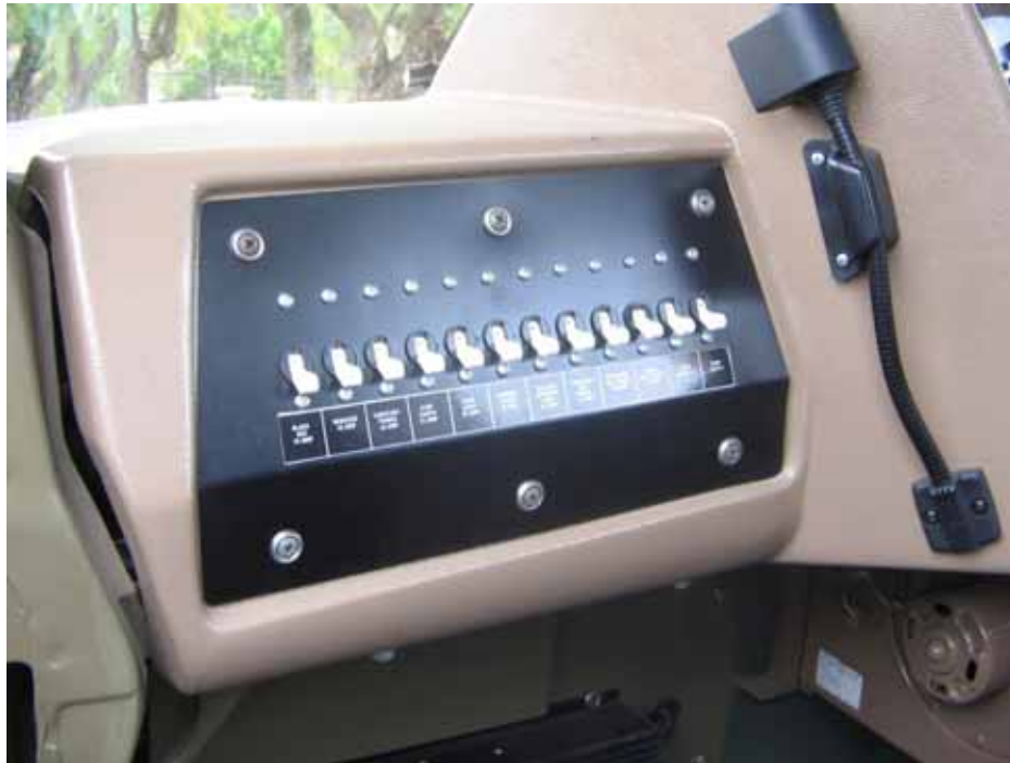
Figure 5 Completed Modified Circuit Breaker Board
