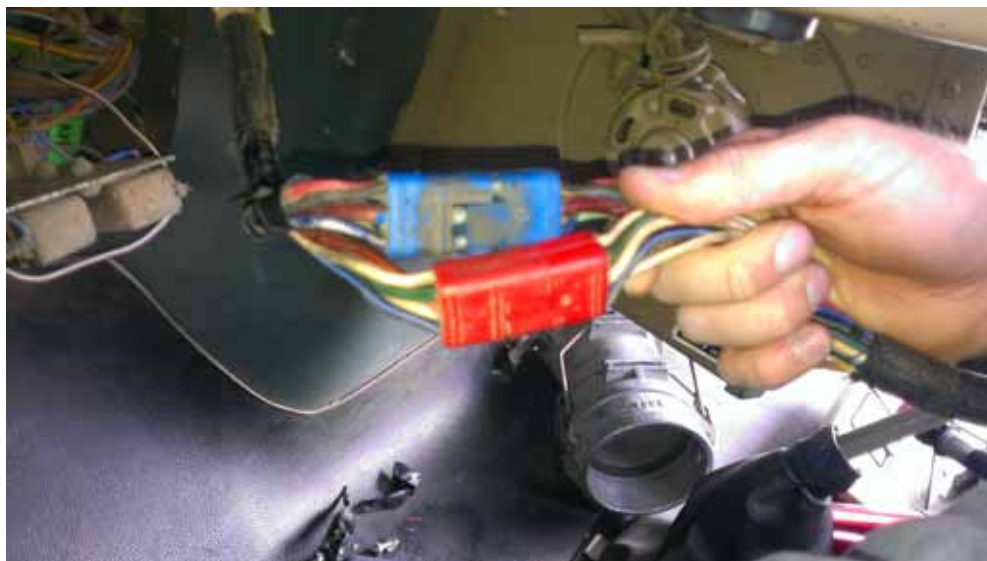
Figure 2 Existing Wiring To Be Disconnected
