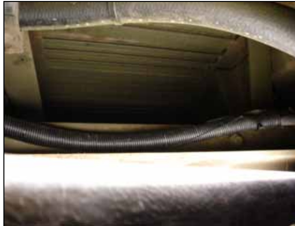
Figure 9 Protective Conduit Installation
