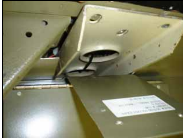
Figure 28 Reinforcement Bracket and Cable Tie Installation
