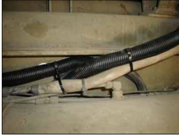
Figure 16 Air Receiver Cable Loop 'Top' Installation
