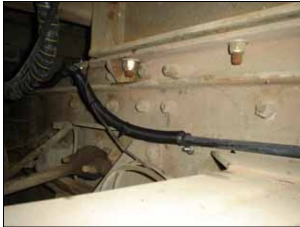
Figure 11 Protective Conduit Installation
