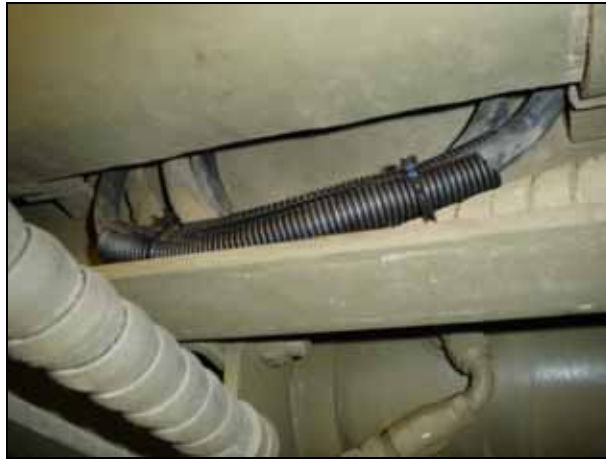
Figure 17 Air Receiver Cable Loop 'Bottom' Installation
