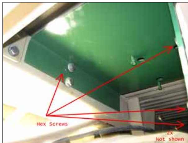
Figure 3 Installation of Plate, Mounting, (W1 Circuit Breaker)
