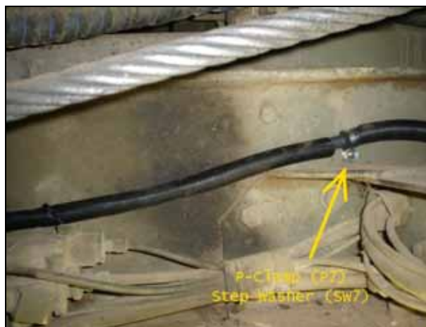
Figure 47 P-Clamp (P7) and Step Washer (SW7) Installation
