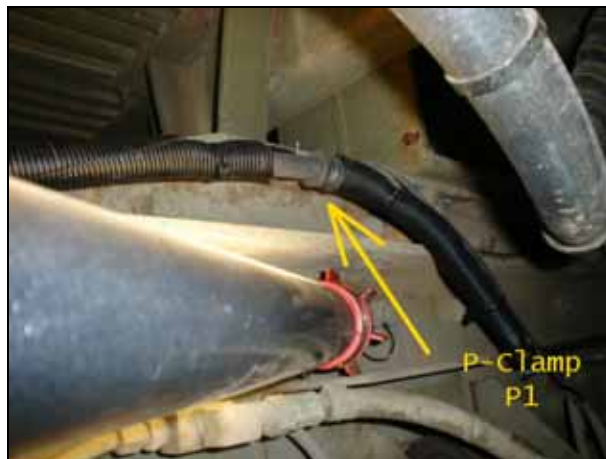
Figure 10 P-Clamp (P1) Installation
