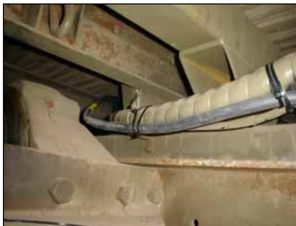
Figure 7 Cable-Tie Fastening
