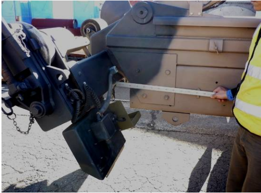
Figure 28 Rear Trestle to Chassis Position
