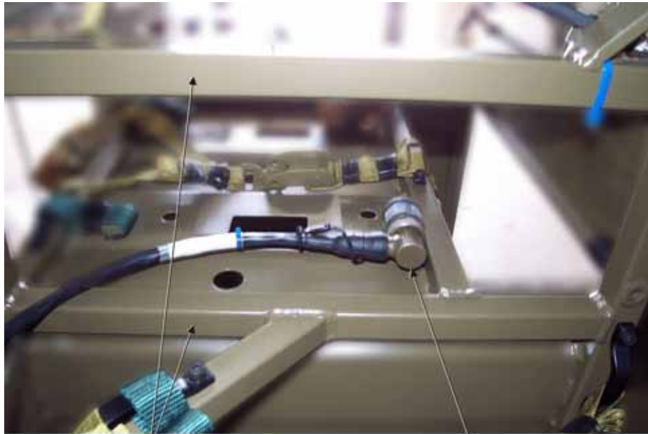
RSU Frame Cable, Vehicle Power, Right Angle Connector Figure 12 Vehicle Power Cable at the RSU Frame
